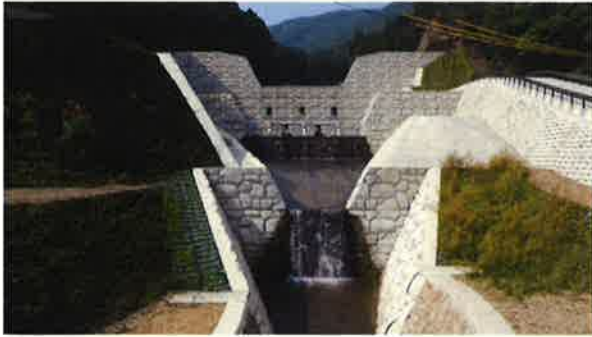
Fig.7 Disaster prevention works of the Nachi-River basin
