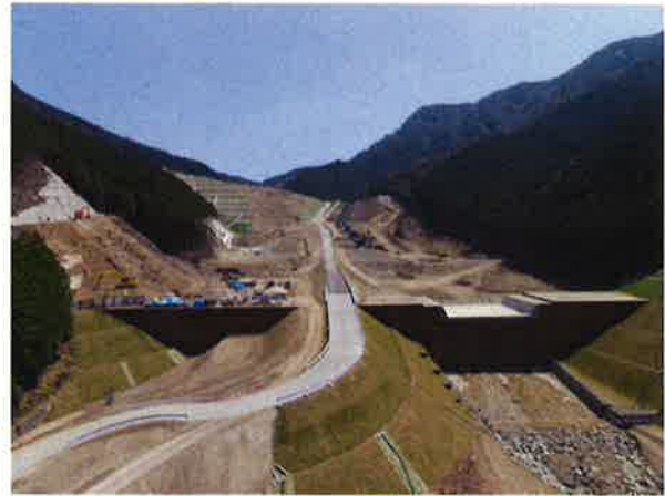
Fig.5 Disaster prevention works of the Iya area
