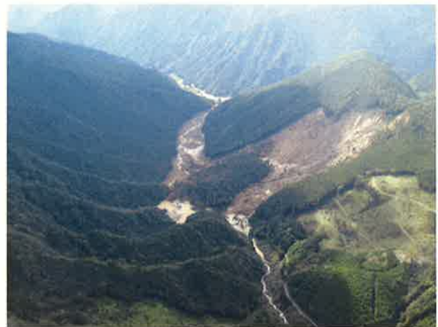
Fig.3 Damage situation of the Iya area
