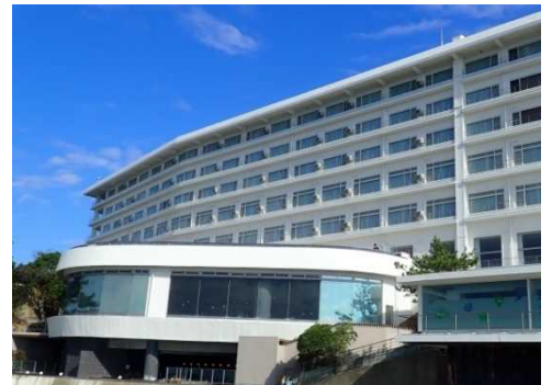
SHIRAHAMA KEY TERRACE HOTEL SEAMORE (耐震改修後)
